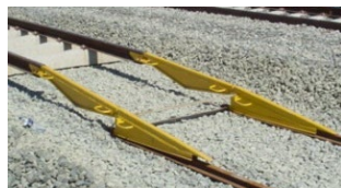
Longitudinal laying with temporary track (VPR)
