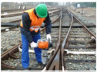
Unscrewing of the most recalcitrant elements of the track
